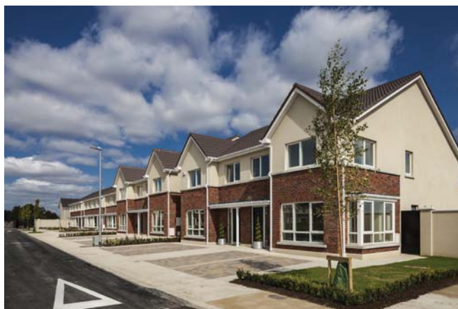
Park Developments Group new energy efficient A2/A3 rated houses at Hamilton Park, Castleknock, Dublin, benefit from Klik heating system
