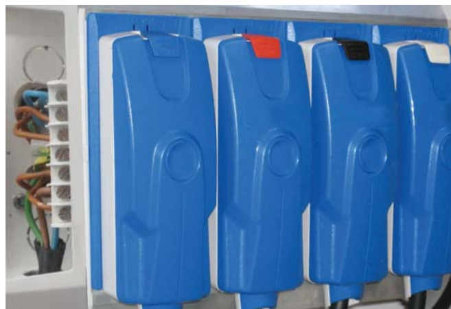
Zone heating system with Klik Heating Box
