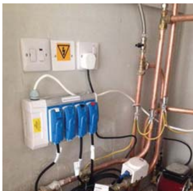
Installation of Klik heating system
